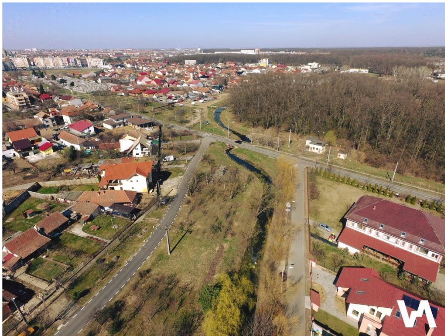
Fig. 7 – Behela undercrossing Ghirodei Alley [23]
